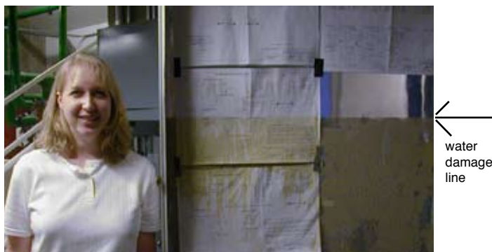
The water level in the mechanical room that serves LCB and the Math Center reached approximately five feet!
